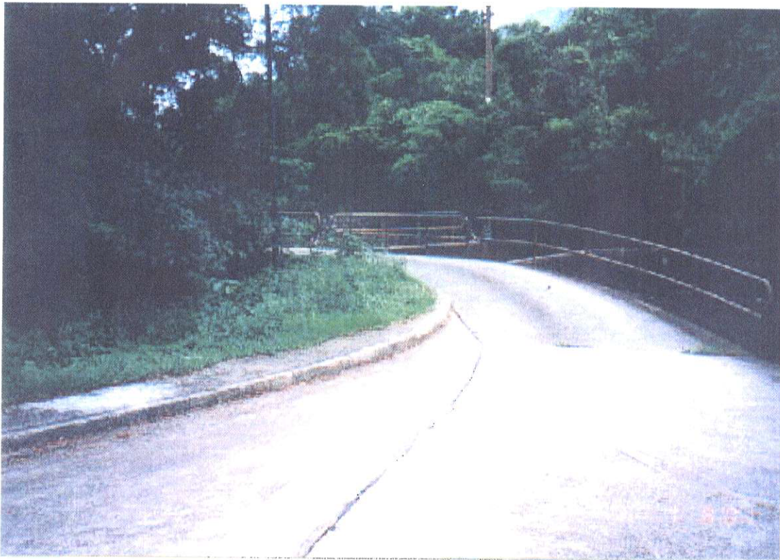
Photograph 11 : Access Road to Site
