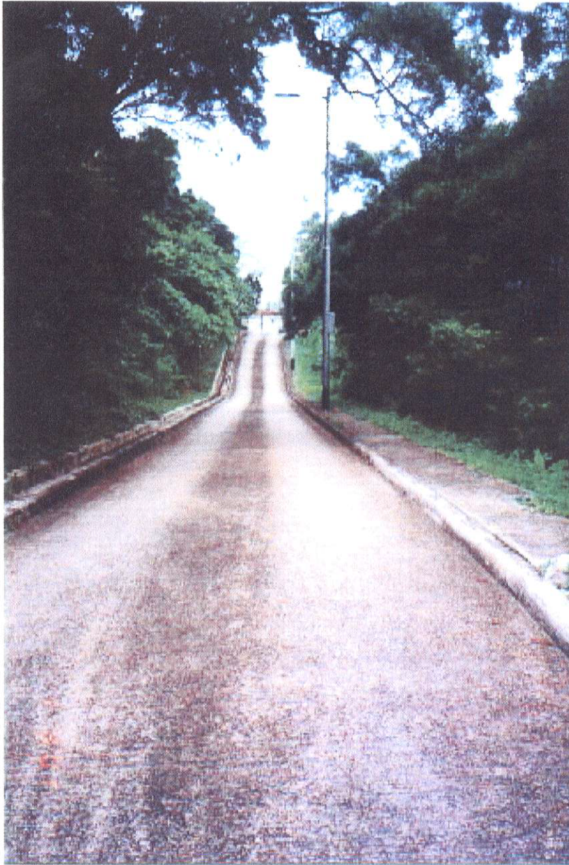
Photograph 13 : Access Road to Site (Section near to WTW after turn off from Catchwater)
