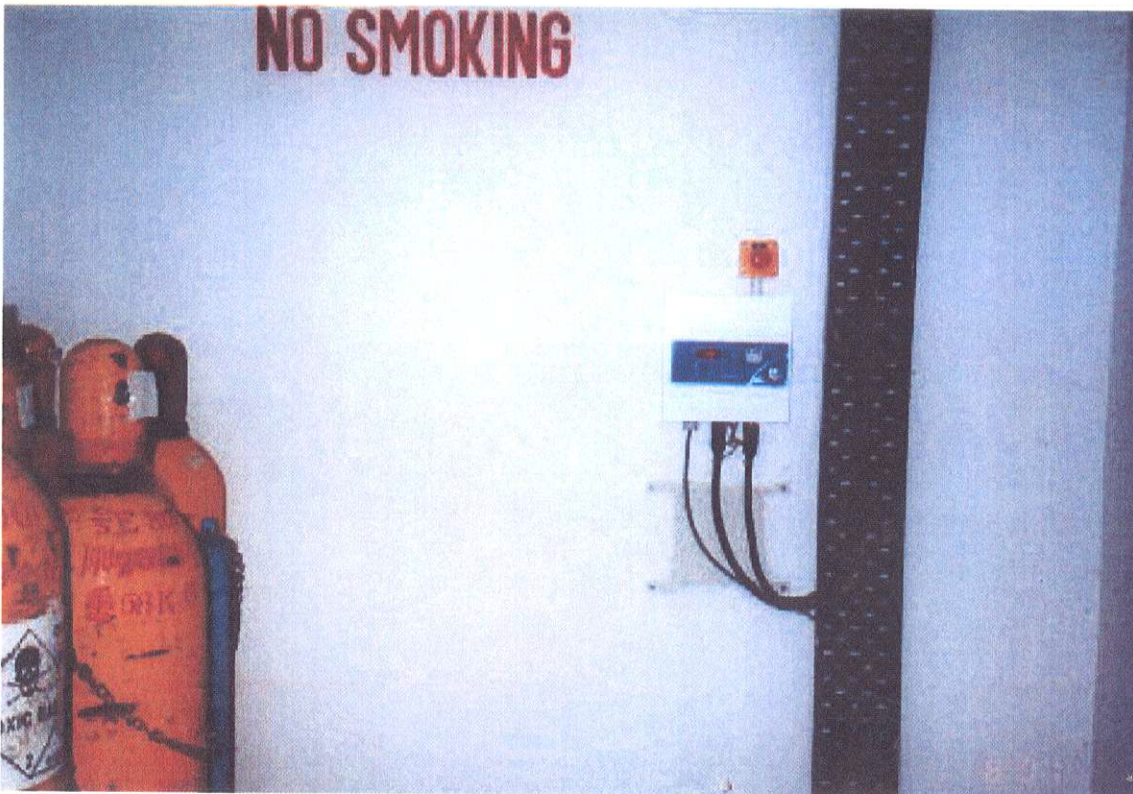
Photograph 6 : Chlorine Gas Detector in Village Chlorine Store
